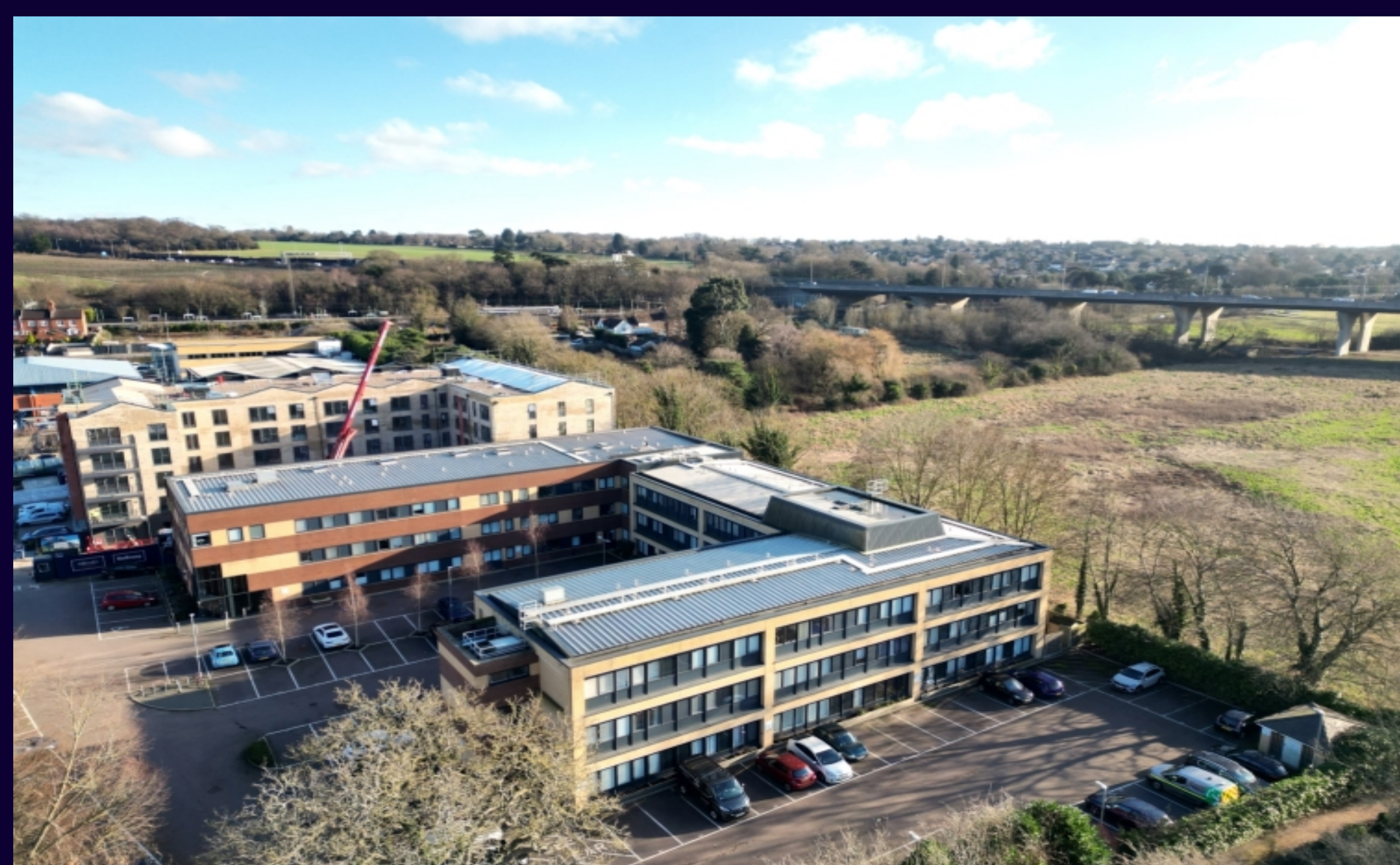
Pinnacle House, Kings Langley, Hertfordshire, WD4 8FW
